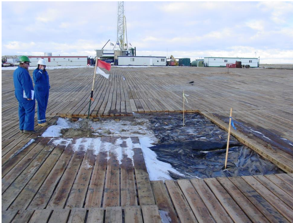
Figure 2. Drill pad constructed with oak mats. Red and white flag denotes drill hole location.
