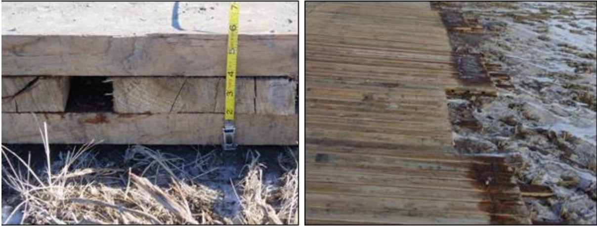
Figure 1. Side view of oak mat illustrating three-ply construction and plank spacing (left photo), and oak mat tongue-and-groove connectors (right photo).
