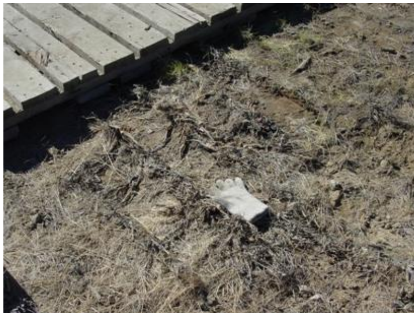
Figure 3. Close-up of ground surface following oak mat removal.
