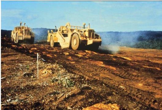
Figure 1: Topsoil stripping operations
