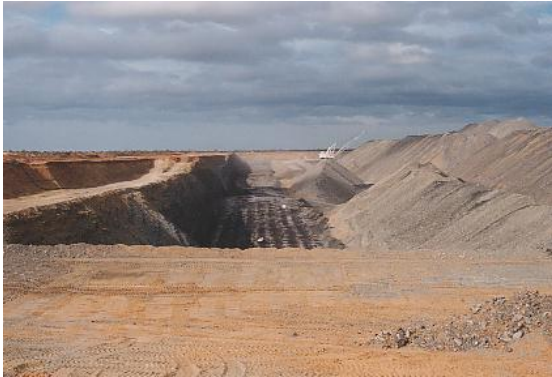
Figure 5: Removing overburden and constructing spoil piles
