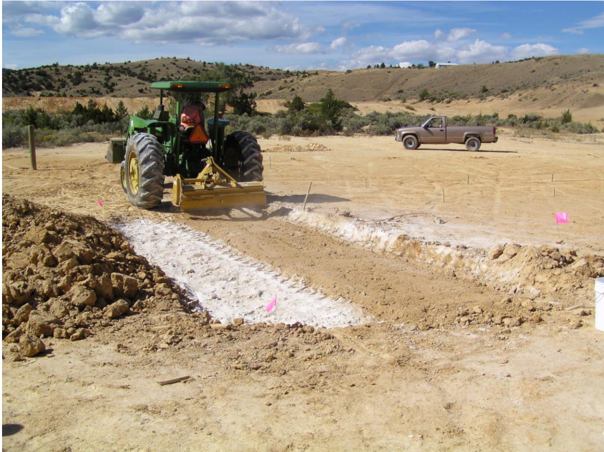
Figure 3. Incorporating lime amendments into an experimental plot at the Keating Tailings, summer 2003.
