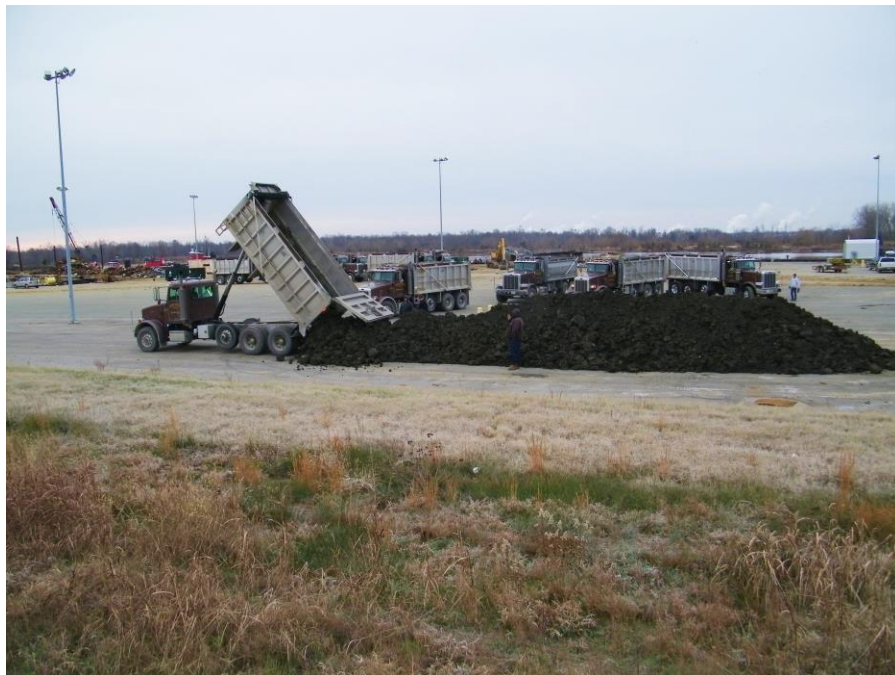
Figure 1. Maryland Port Administration Cox Creek Facility dredge material being placed at Port Tobacco, Shirley Plantation, Charles City, VA, in November of 2009. The materials were immediately covered with a tarp to limit rainfall additions and oxidation.
