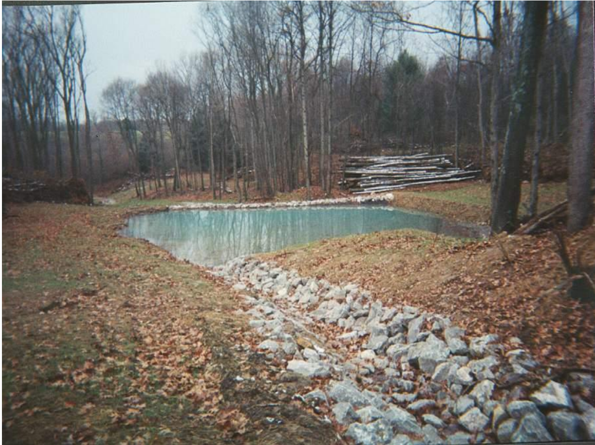
Figure 2. Leach bed #1 and OLC #1 at the McCarty Highwall AMD treatment project
