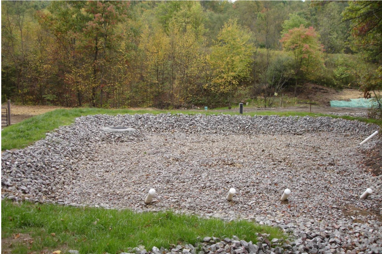
Figure 4. Steel slag leach bed under construction at the DeAntonis project site.
