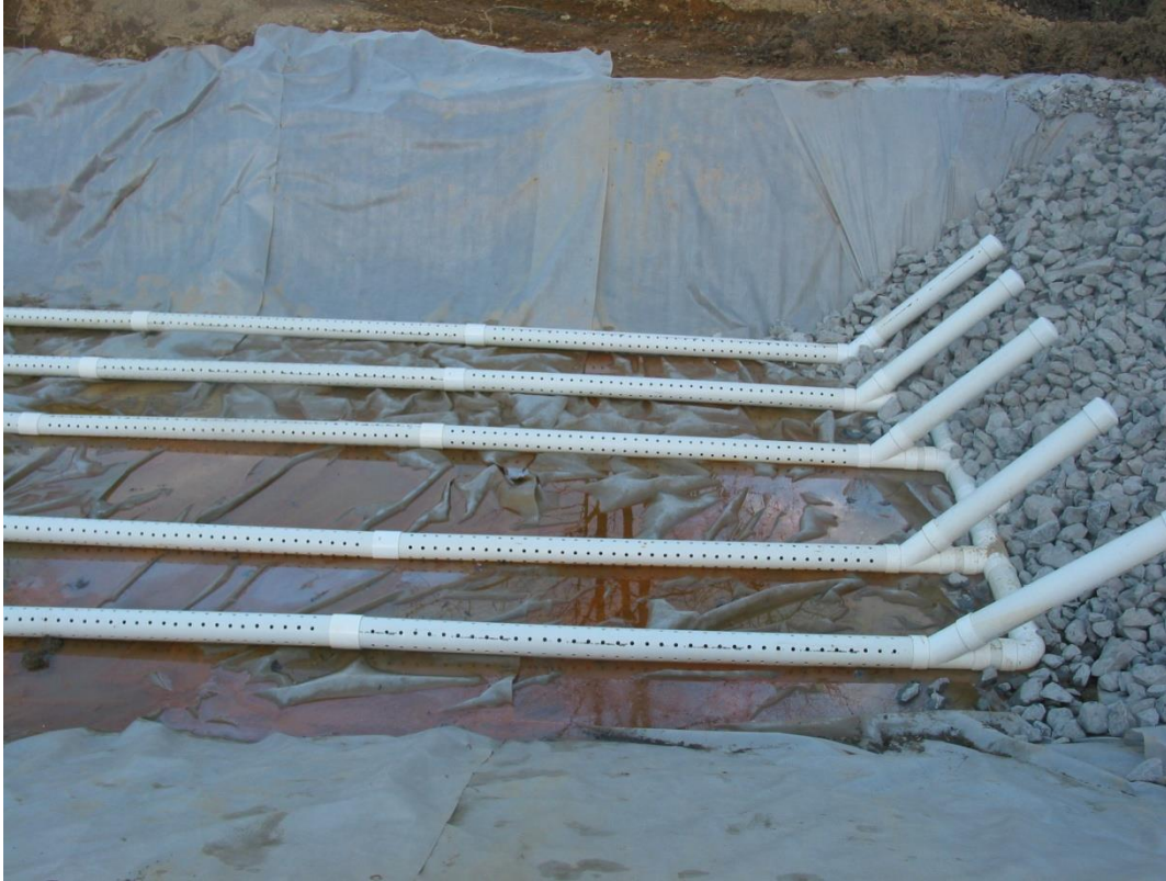
Figure 6. Steel slag leach bed under construction at the Muzzleloader Club site.
