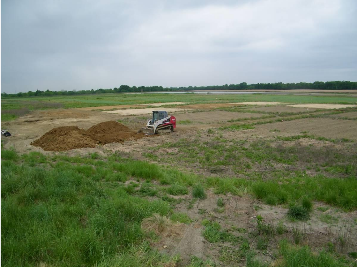
Figure 3. Installation of main treatments at the Earle Soil Amendment Crop Plot Experiment, Charles City, VA. Photo taken from southeast corner of plots.
