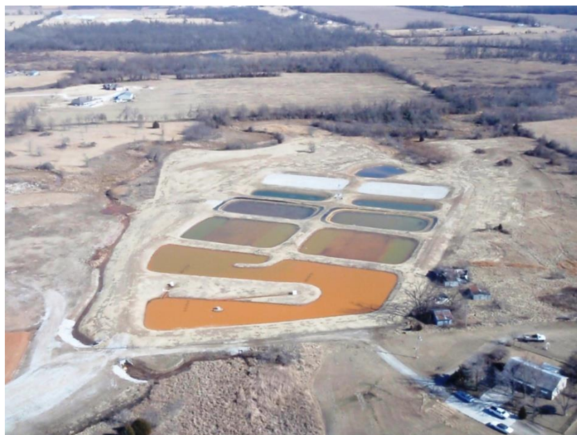
Figure 1. Aerial photograph of Mayer Ranch passive treatment system, NE Oklahoma (pH = 6)
