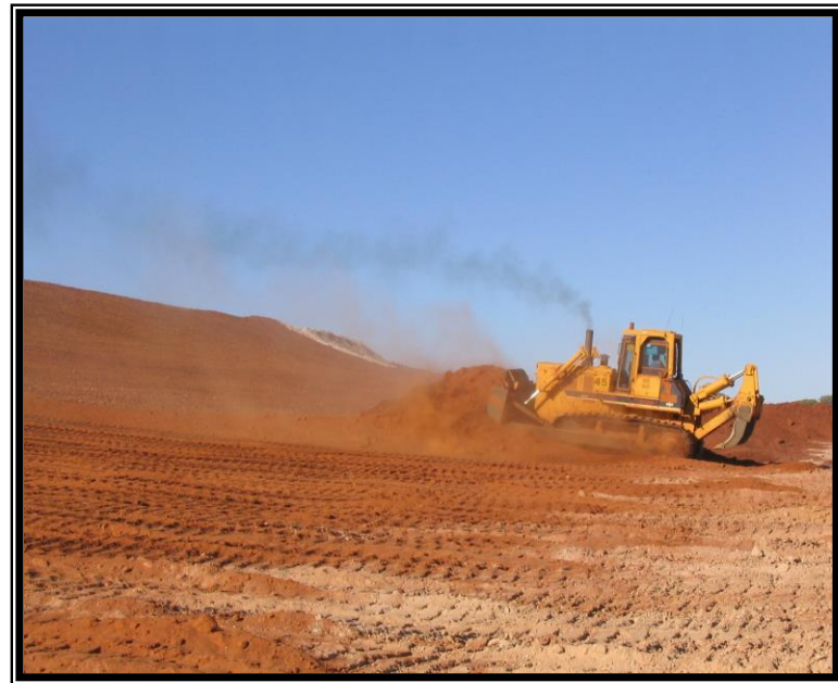
Plate 6 Fine topsoil placed over laterite
