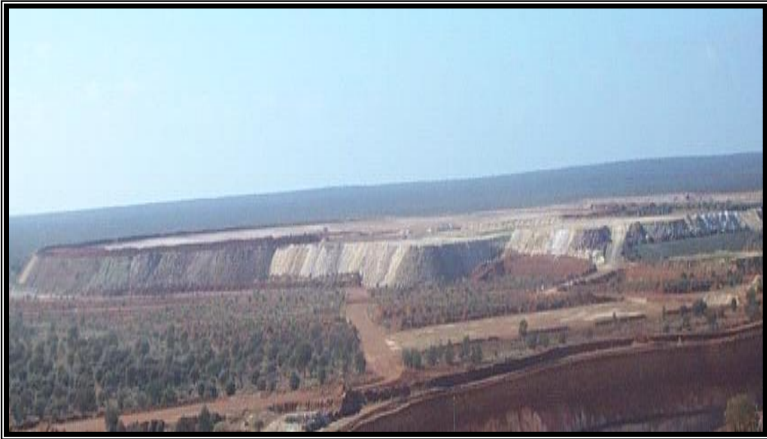
Plate 8 TSF4 Before Rehabilitation Works
