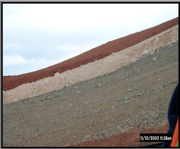
Plate 3 Laterite placed over oxide layer on PAF slopes
