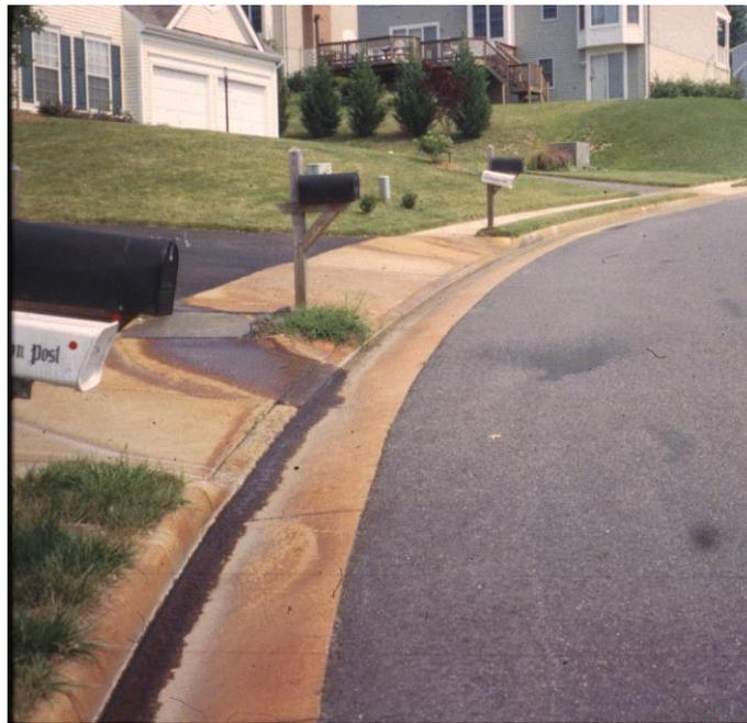
Figure 4. Acid drainage from the Quantico slate in Stafford, Virginia (see also Fig. 1), has caused extensive iron staining along curbs and sidewalks through the Hampton Oaks subdivision. Also, concrete etching occurs when acid drainage “dissolves” out the cement, deteriorating the concrete. Homeowners in this neighborhood apply the equivalent of 2 Mg agricultural lime per hectare per month to maintain soil pH above 5.5.
