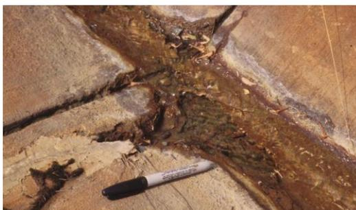
Figure 1. Acid drainage from the Quantico slate Stafford, Virginia, (see also Fig. 4) has caused extensive iron staining and concrete etching along the curbs and sidewalks of the Hampton Oaks subdivision.
