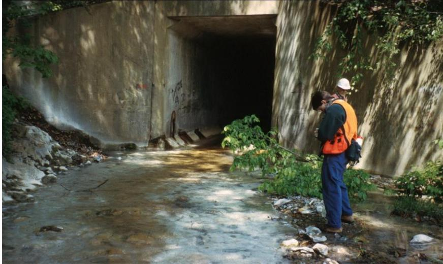
Figure 3. Acid drainage from the Millboro shale, exposed along I-64 in Clifton Forge, has contaminated this stream. The pH of water samples from the downstream end of the culvert has ranged from 2.9 to 7.1. Iron and aluminum precipitates coat the streambed, and concrete joints within the culvert have been degraded.
