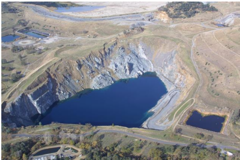
Figure 1. An open pit gold mine with slopes that were stable long enough to complete mining, but failed soon after mining was completed.
