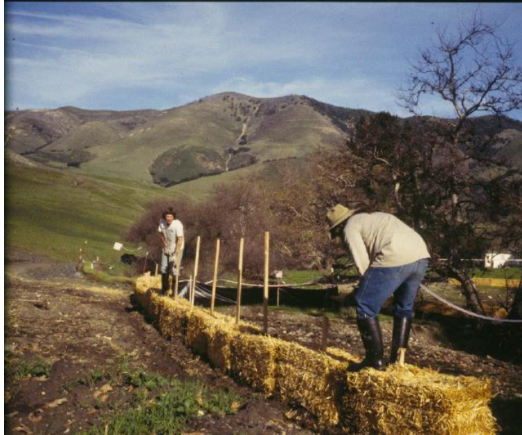
Figure 5. Straw bails and geotextiles being used for temporary erosion control.
