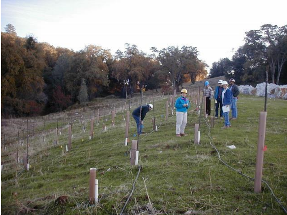
Figure 2. A recently revegetated fill slope with plant protection and irrigation temporarily in place until performance criteria are met.
