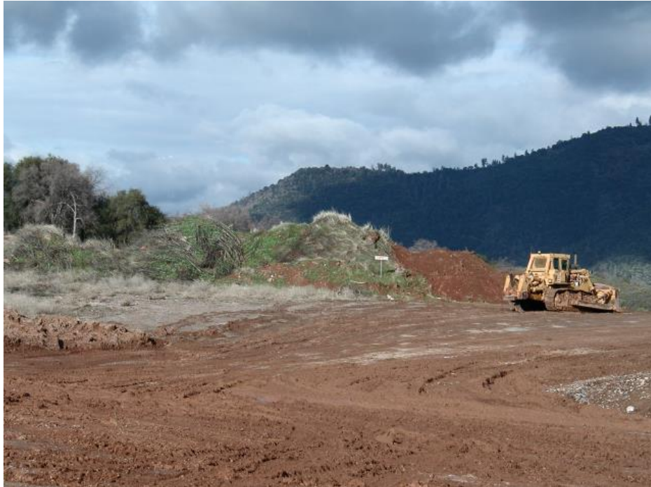
Figure 3. Stockpiled topsoil being redistributed in preparation for planting.
