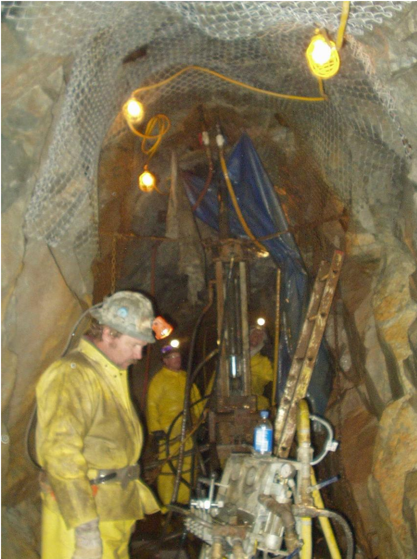
Figure 21. Waternight plug station with Hagby core drill drilling borehole to surface
