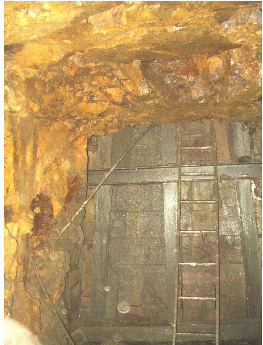
Figure 22. I-beam and Timber Constructed Bulkhead for Plug Station
