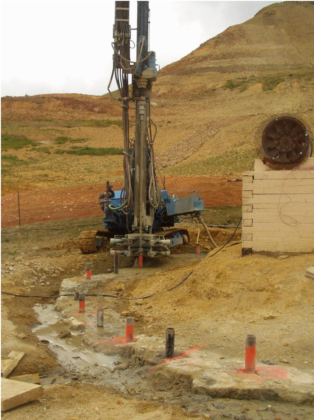
Figure 15. Rotary drilling primary (Red) and secondary drill holes into bedrock.
