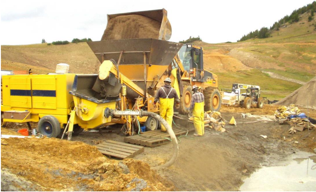
Figure 17. Continuous 15 cubic meter/hour concrete batch plant at the Como Raise.
