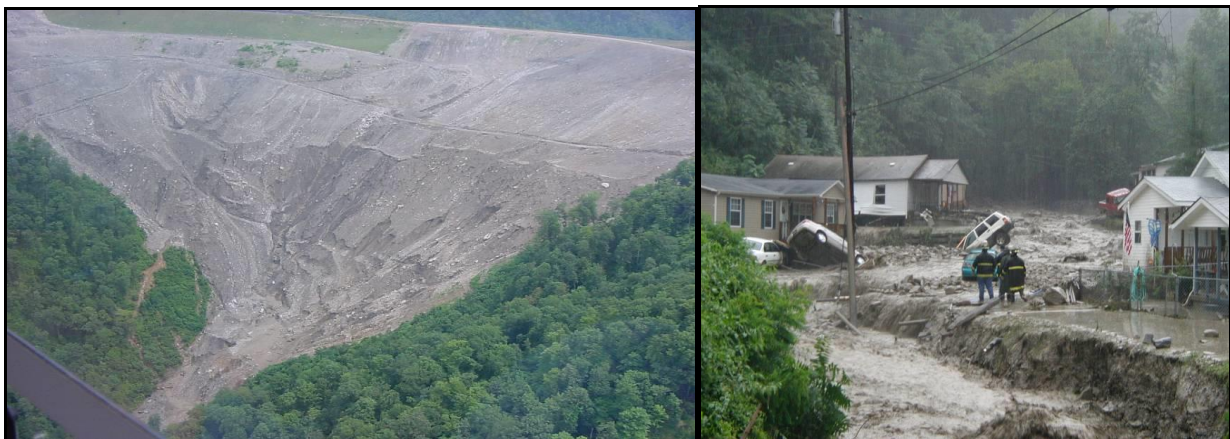
Figure 5: Lyburn flood; (left) erosion and sloughing on the outslope of the durable rock fill following storm event; (right) property damages downstream of the fill.
