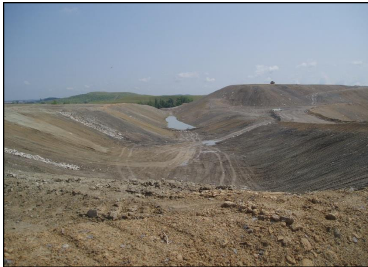
Figure 8: Backfill grading to construct a cattle watering hole on a mountaintop mining site being reclaimed.
