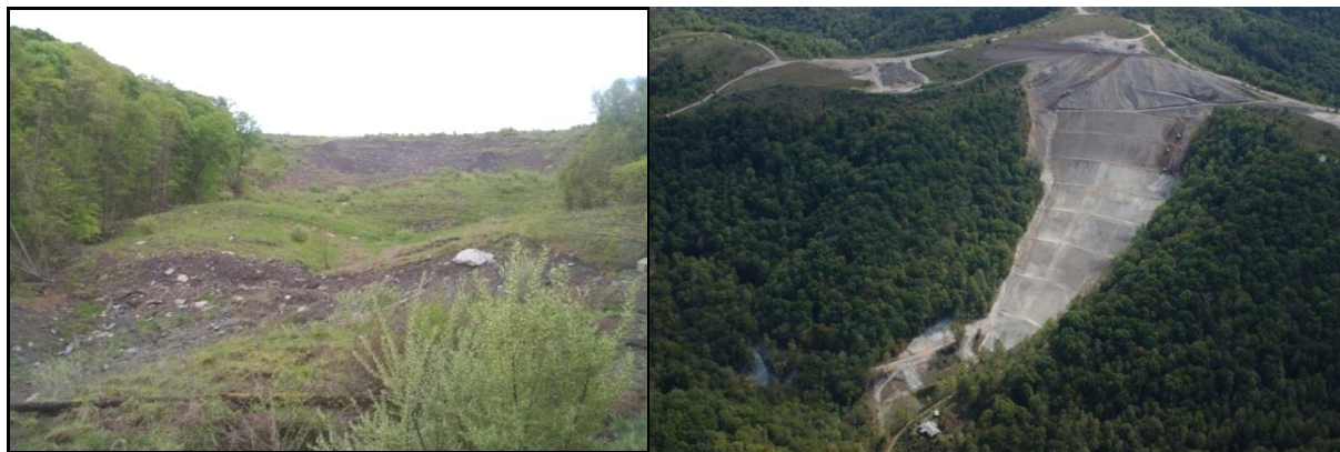
Figure 3: HNR durable rock fill in eastern Kentucky; (left) general view of landslide looking upslope from toe; (right) aerial view of fill during the post-landslide remediation.
