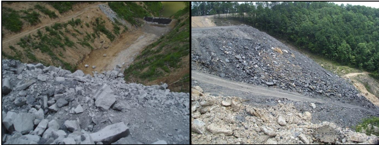
Figure 4: Gravity segregation of durable rock fill underdrains; (left) effective underdrain formation with durable sandstone boulders; (right) ineffective underdrain formation with “durable” shale fragments.
