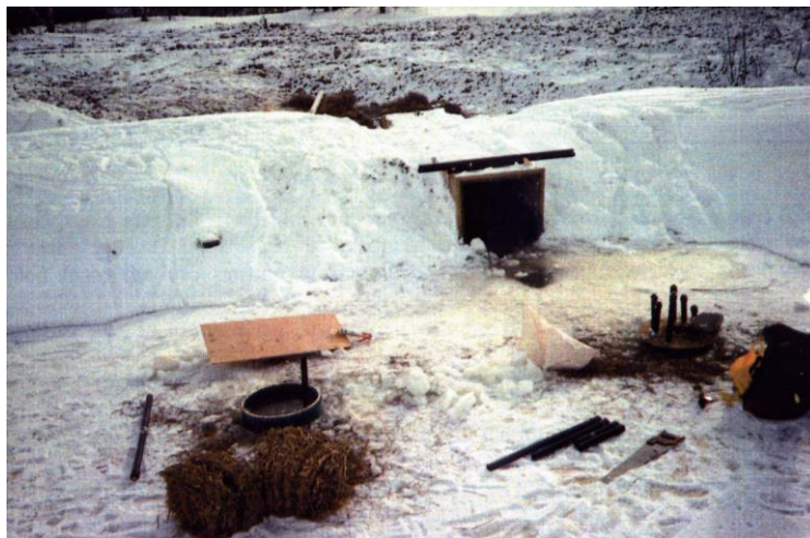
Figure 3a: Arumator under construction.
