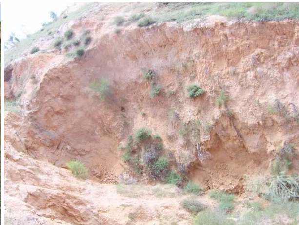
Figure 2. Subsidence and erosion in loess area
