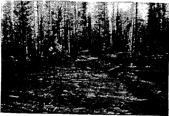
Figure 13. Bulldozer fireline prior to rehabilitation. (Bundros)
