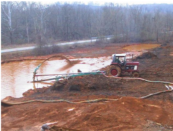
Figure 4. Sludge removal with a tractor pump.
