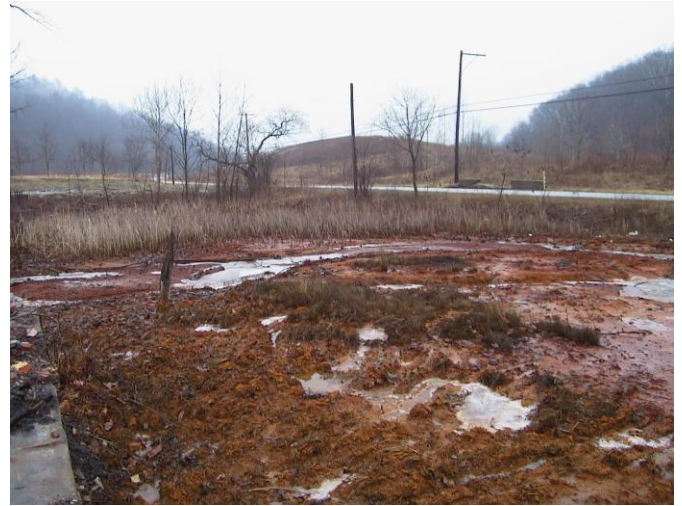
Figure 2. The sludge-filled channel before processing activities.
