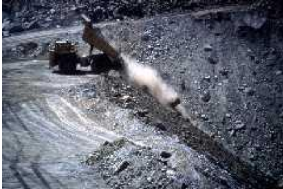
Figure 3: Typical End-Dumping Placement Methods
