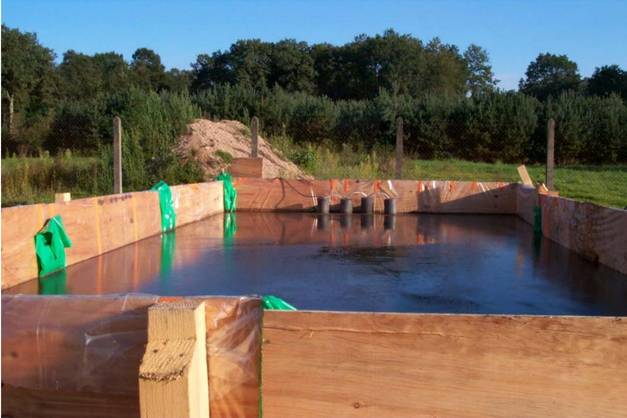
Figure 6. Treatment basin containing 350 tons of sludge contaminated with mercury from dental amalgams, Montluçon, France.
