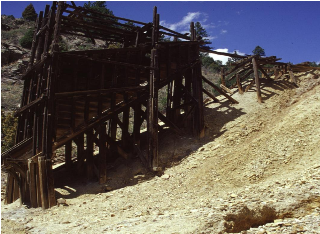
Figure 1. Ore takeout at the Rattler Site in May 2004.
