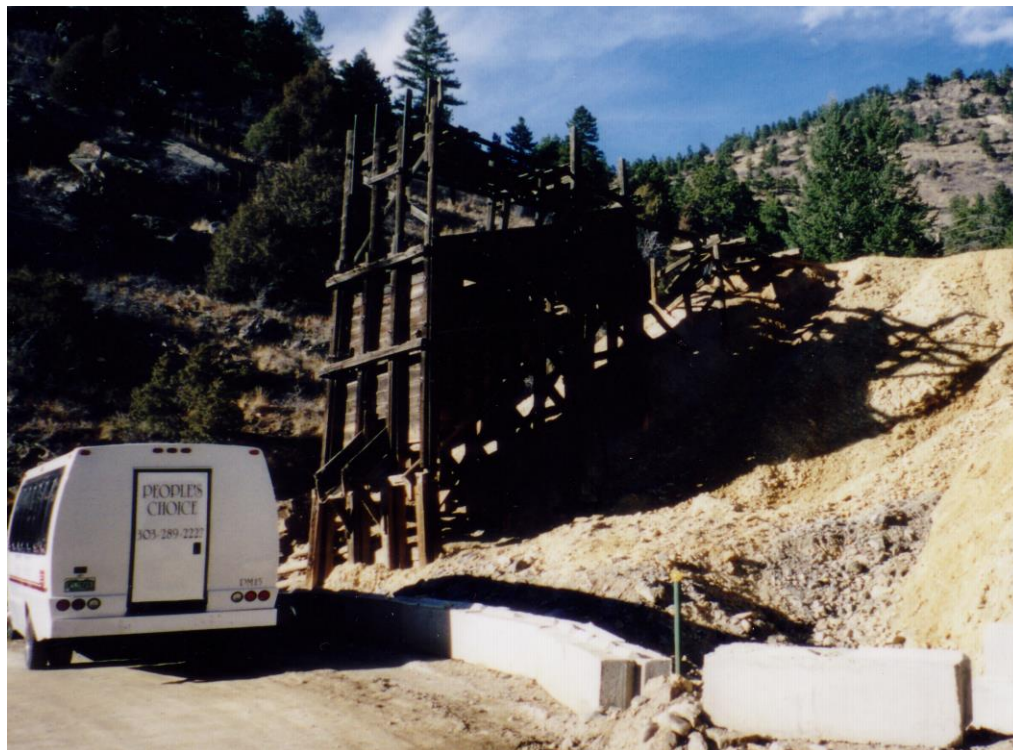
Figure 2. Ore takeout at the Rattler site in November 2004 after the large rain event (Notice the barriers that were installed after the event to push back and retain washed out materials from blocking the road).
