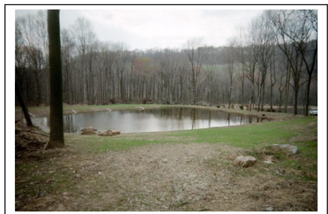
Figure 3. Sulfate Reducing Bioreactor
