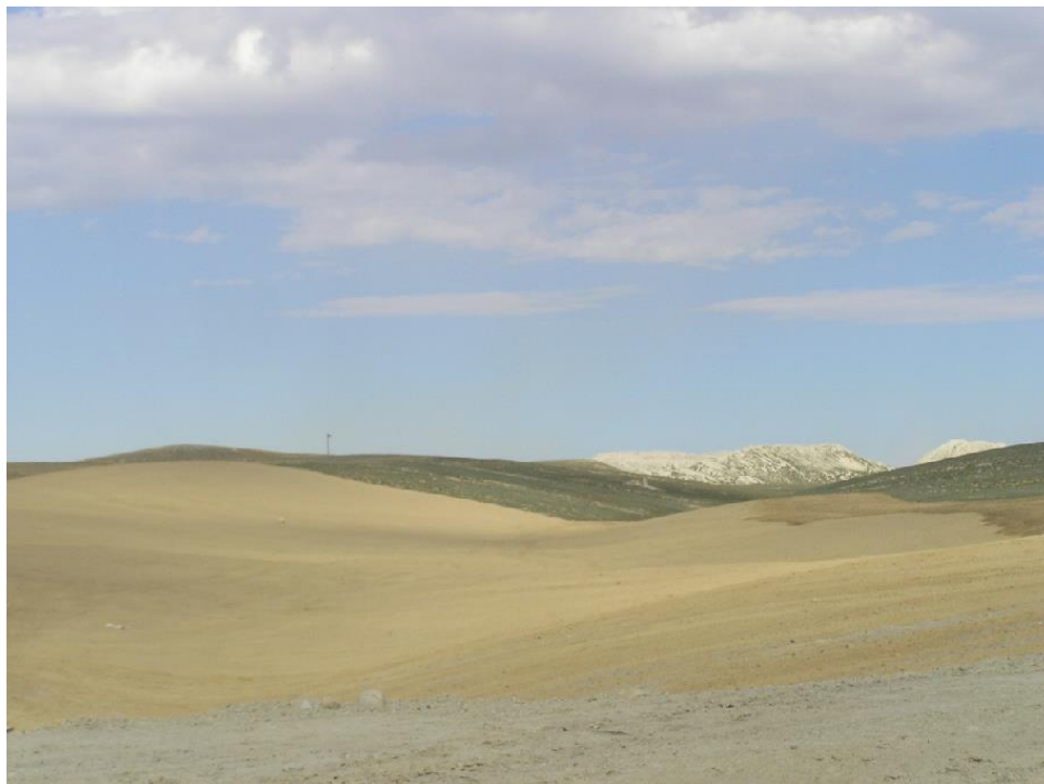
Figure 5. Finished Grading (Fall 2006)
