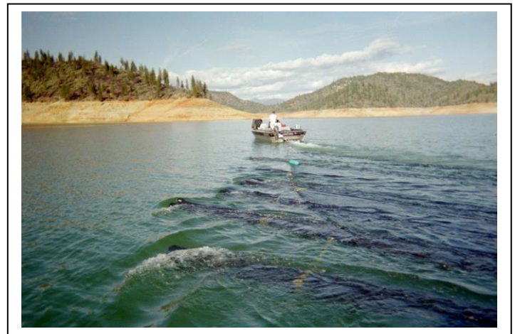
Figure 8. Transport of 6-inch HDPE pipe across Lake Shasta
