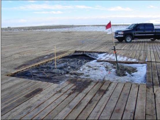
Figure 1. View of a drill pad constructed with oak mats.
