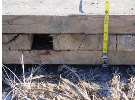
Figure 2. Cross section of an oak mat constructed from individual oak boards.
