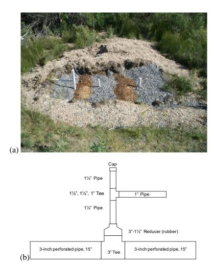
Figure 3. Second pilot-scale biocell. (a) image form construction. (b) effluent piping.
