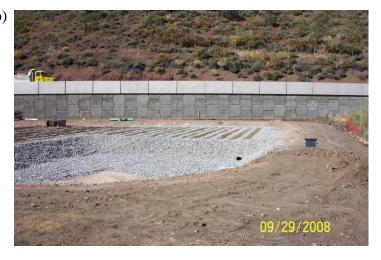
Figure 5. Biocell construction. (a) Placement of gravel and substrate in biocell. (b) View of construction showing effluent pond in foreground. Dark box atop berm at right is top of the water control structure.
