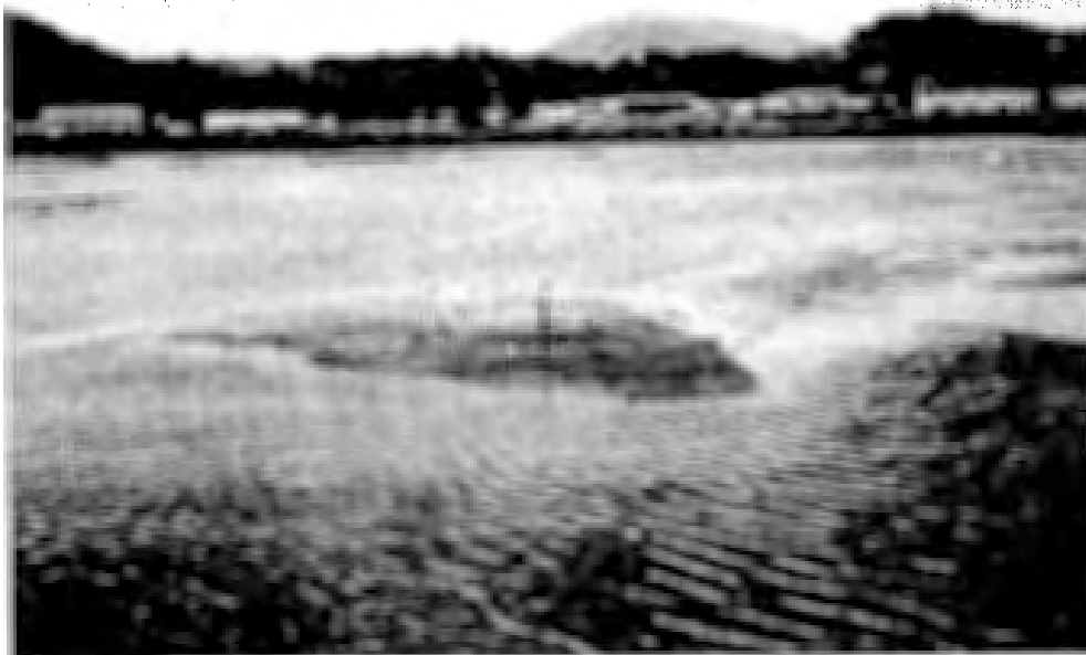
Figure 5. Sedimentation of detention basin
