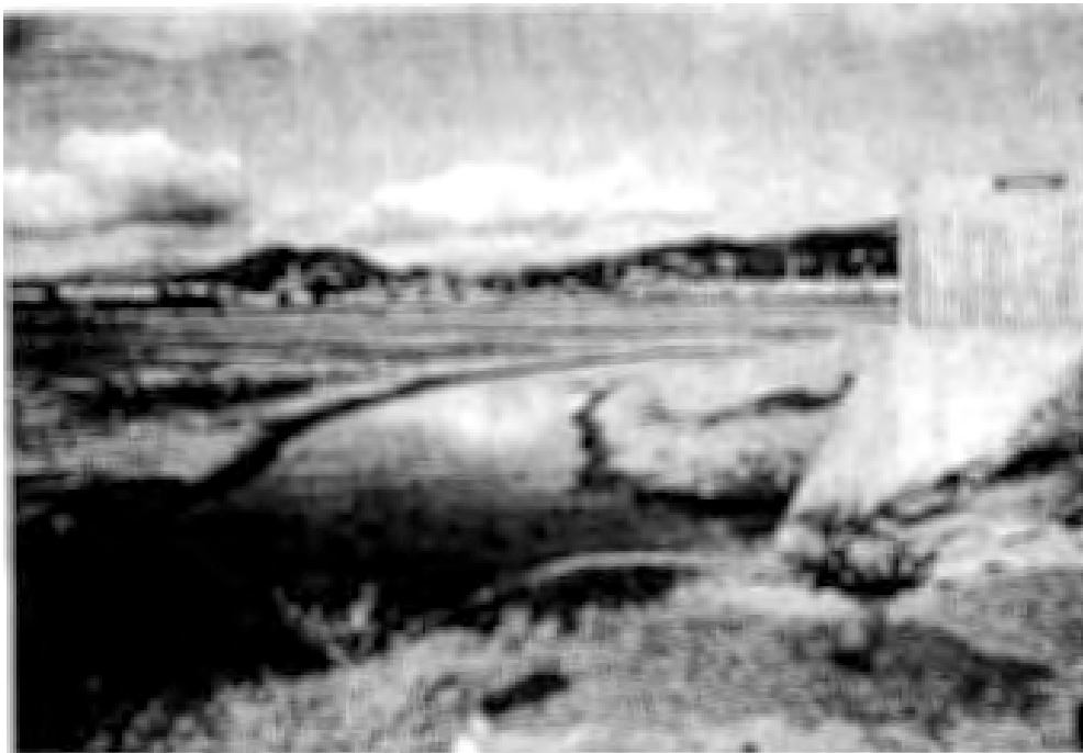
Figure 9. Pumpstation showing inlet canal
