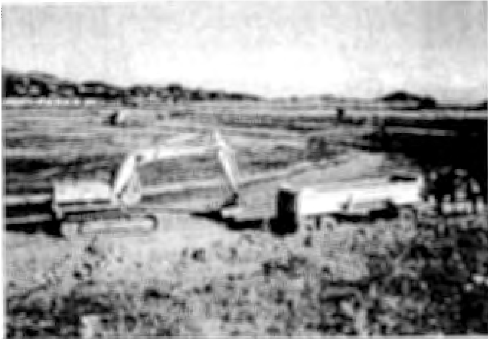
Figure 8. Excavation of detention basin inlet canal showing pump station in background
