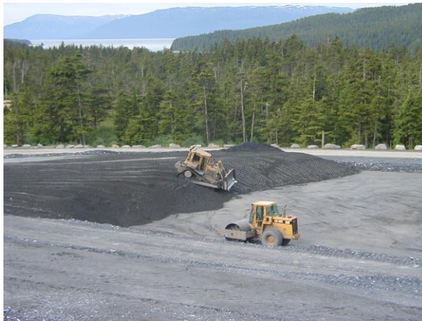
Figure 4. D6 CAT spreading tailings. Vibratory roller on compacted lift in foreground
