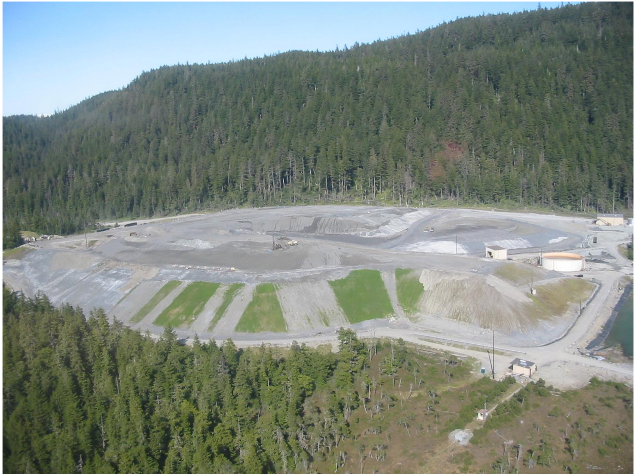
Figure 2. Aerial photograph of the Greens Creek dry-stack tailings pile in May 2005.
