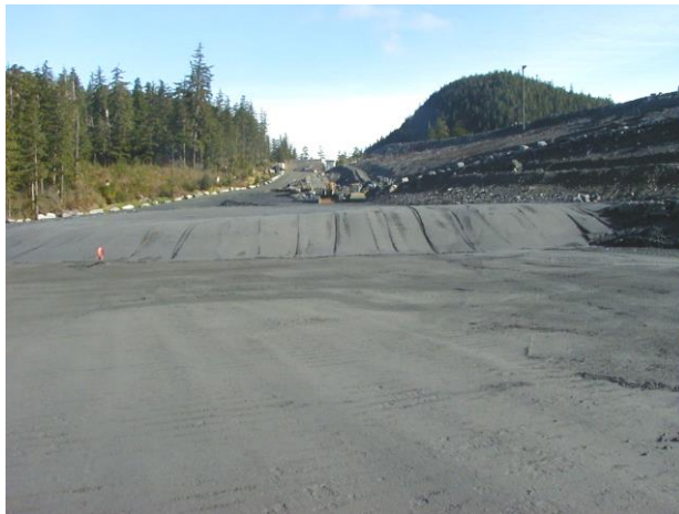
Figure 5. Roller-compacted tailings.
