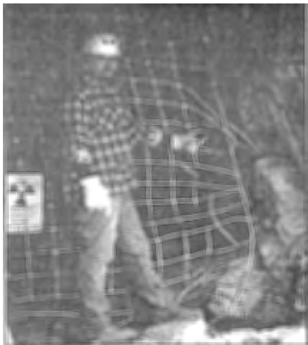
Figure 6. Cable Net closure in Laythrop Canyon Project, 1990.
