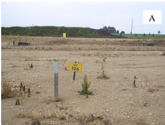
Figure 6. A, Site stripped of topsoil, stockpile visible in distance, as part of suburban development in Northern Illinois; B, sod laid directly on graded subsoil in new Central Illinois suburban development.
