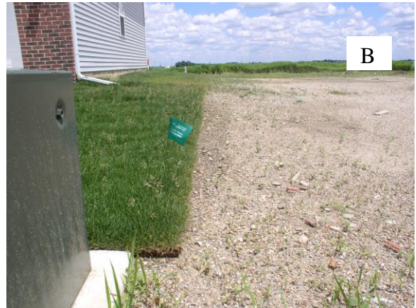
Figure 6. A, Site stripped of topsoil, stockpile visible in distance, as part of suburban development in Northern Illinois; B, sod laid directly on graded subsoil in new Central Illinois suburban development.
