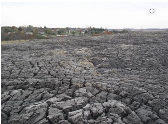
Figure 4. Sediment application as a topsoil substitute at Pekin IL Landfill: A, clam shell bucket loading Peoria Lake sediment onto a deck barge; B, stockpiling sediment on top of Pekin Landfill clay cap; C, drying sediment one month after placement; D, volunteer vegetation thriving on sediment, unvegetated foreground is landfill clay cap, one year later.
