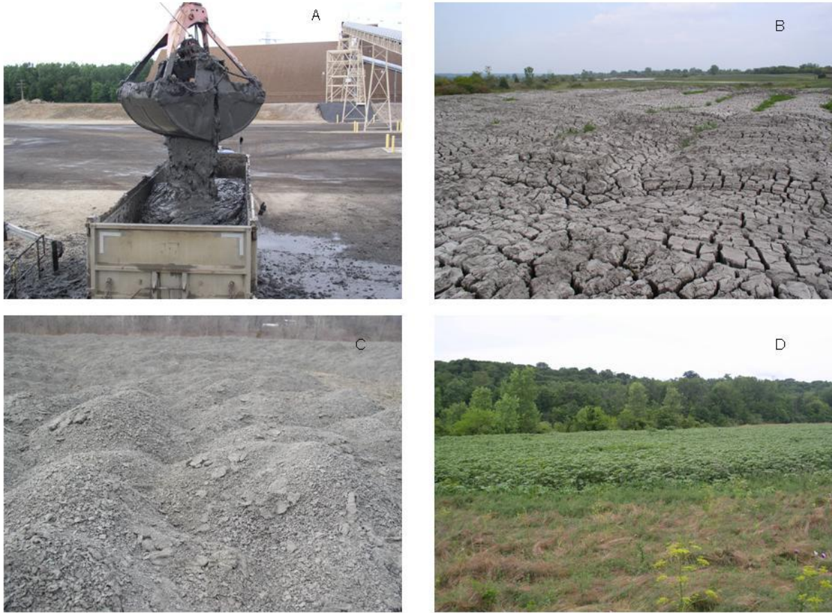
Figure 5. A, Truck receiving sediment from barge for transport to Banner Marsh pre-law strip mine area; B, Sediment drying one month after placement; C, frost shattered sediment polygons the following spring; D, Planting of sunflowers thriving on sediments after tillage, foreground is untreated.
