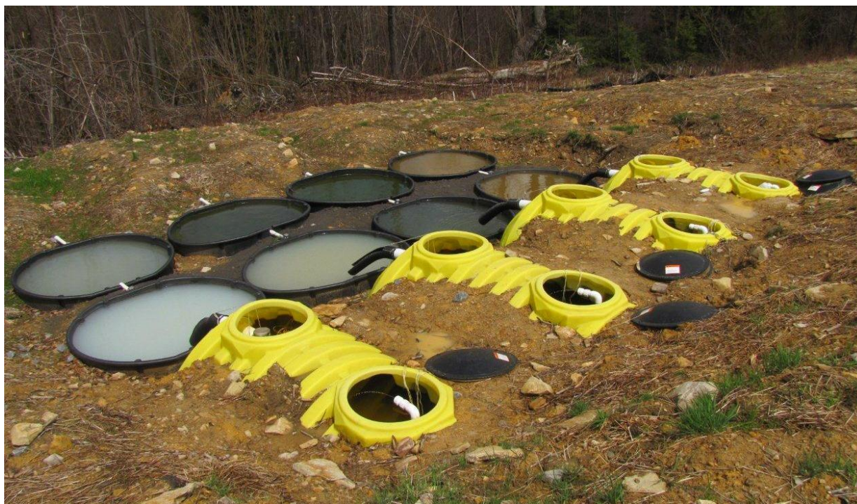
Figure 4. Pilot-scale VFPs and subsequent aerobic settling ponds installed to treat MIW at the Klondike-1 field site. Photo taken on April 26, 2011, by Brandon Diehl, Foundation for Pennsylvania Watersheds.
