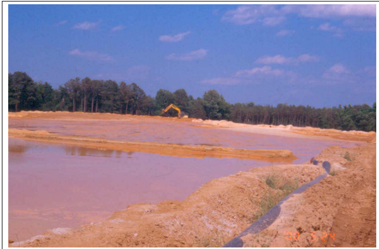
Figure 4. Mining pit being backfilled with mixed tailings and slimes at Old Hickory. The light colored materials in the background are sandy tailings while finer-textured slimes have migrated to the calmer water environment in the foreground. Recent (post-2000) utilization of internal cross-dikes as seen here has minimized segregation to some extent. Material in the immediate right foreground is topsoil forming an enclosing dike.
