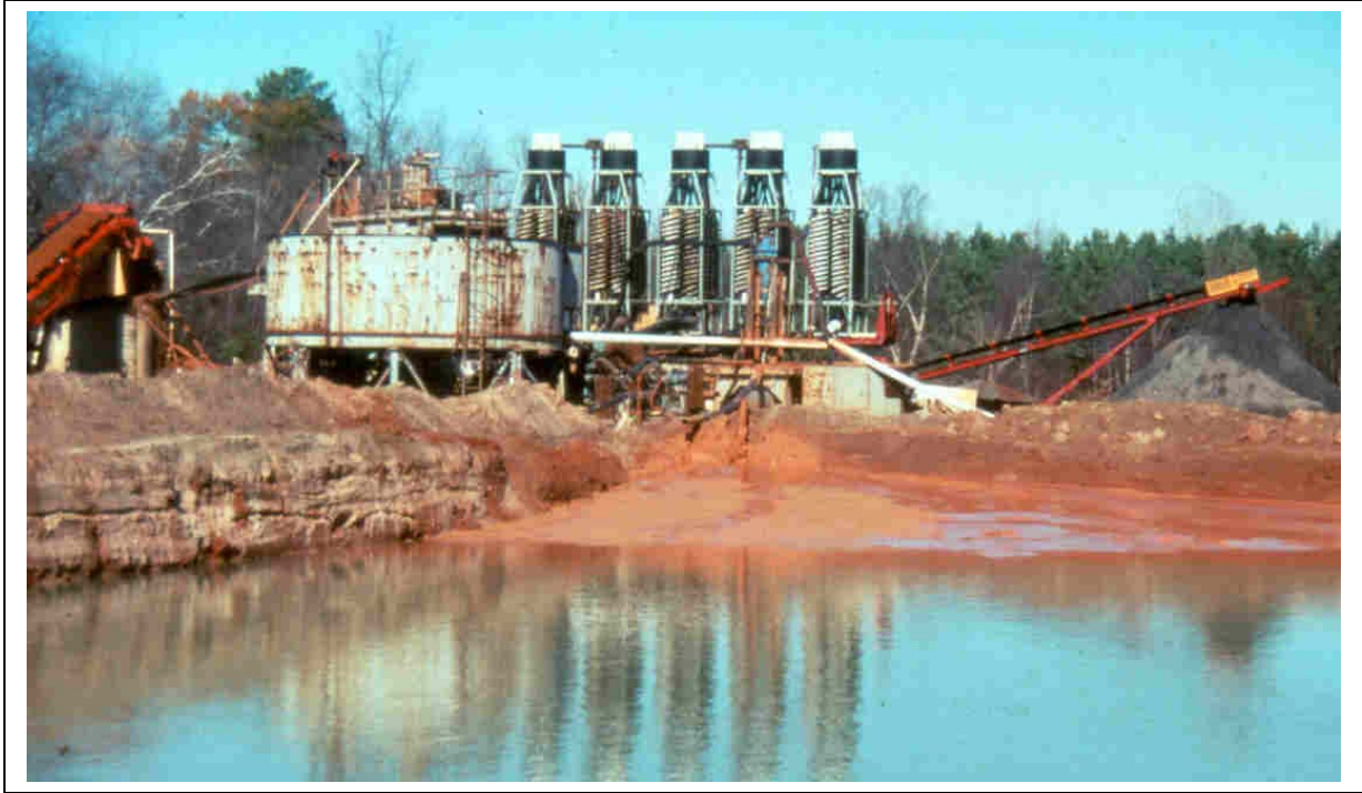
Figure 2. Pilot processing plant and adjacent test pit in 1995. Spirals for sand separation are shown in middle background and the slimes thickener tank is on the left. Mixed tailings and slimes are being deposited in the foreground into one of the three test mining pits.
