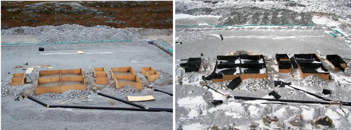
Figure 8. Photo to the left show three lysimeter clusters constructed over the Type III test pad. Loops of wire on the lysimeter pads are heat trace cable. The black 10-inch insulated pipe house the 1.5-inch drainage pipes exiting from each lysimeter. The photo to the right shows a completed cluster lysimeters with an impermeable HDPE liner.
