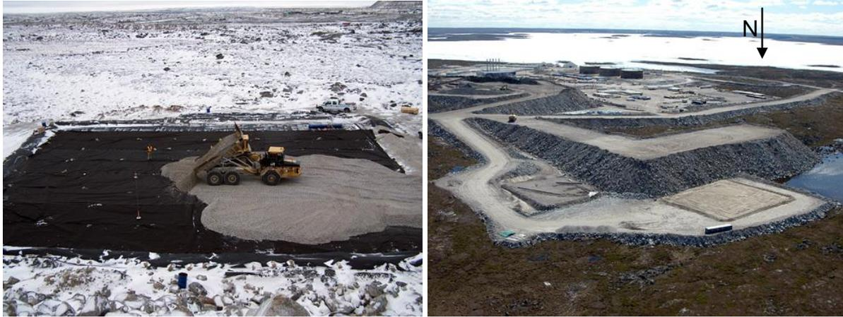
Figure 6. Photo to the left shows crushed rock being place over the impermeable liner of the Type I rock pad. Photo to the right shows the positions of the Type I pad (left) and Type III pad (right). The dimension of each pad is 50 m × 60 m. The L-shaped ramp adjacent to the test pads in the foreground will be used to tip rock onto the pads for construction of the waste rock piles. The arrow to the right of the photo is pointing North.
