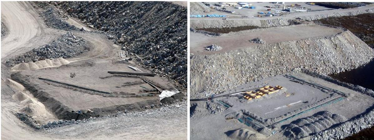
Figure 7. Photo to the left show the basal drainage ditch excavated diagonally across the center of the Type I pad exiting through the SW corner. Photo to the right shows the basal drainage ditches excavated around the perimeter of the Type III pad exiting though the NE and NW corners.
