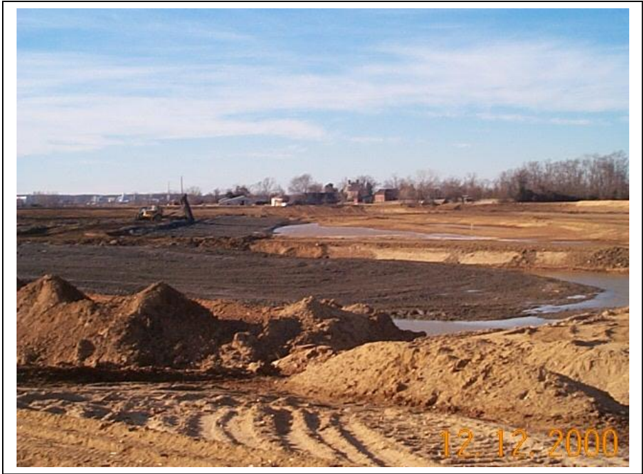
Figure 2. Reduced dredge materials being placed in December 2000. Picture was taken atop enclosing dike looking NW with Shirley Plantation house in background. Agricultural experiments were installed in August 2001 in area immediately to the left of this photograph.
