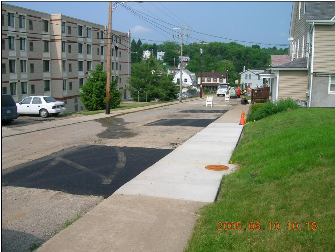
Figure 9. View of the manhole cover of the Early Warning System in the repaired sidewalk. (06/10/05)
