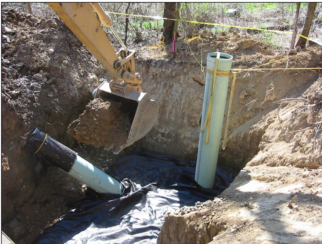
Figure 7. Construction of Secondary Drain. Geotextile used for layer separation of aggregate and backfill. (04/13/05)
