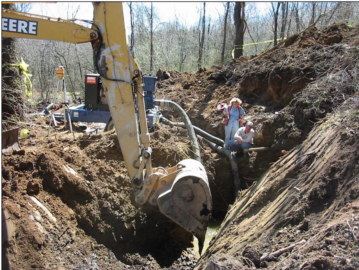
Figure 3. Test pits excavated with pumping conducted to determine favorable locations for Primary and Secondary Drains. (04/08/05)
