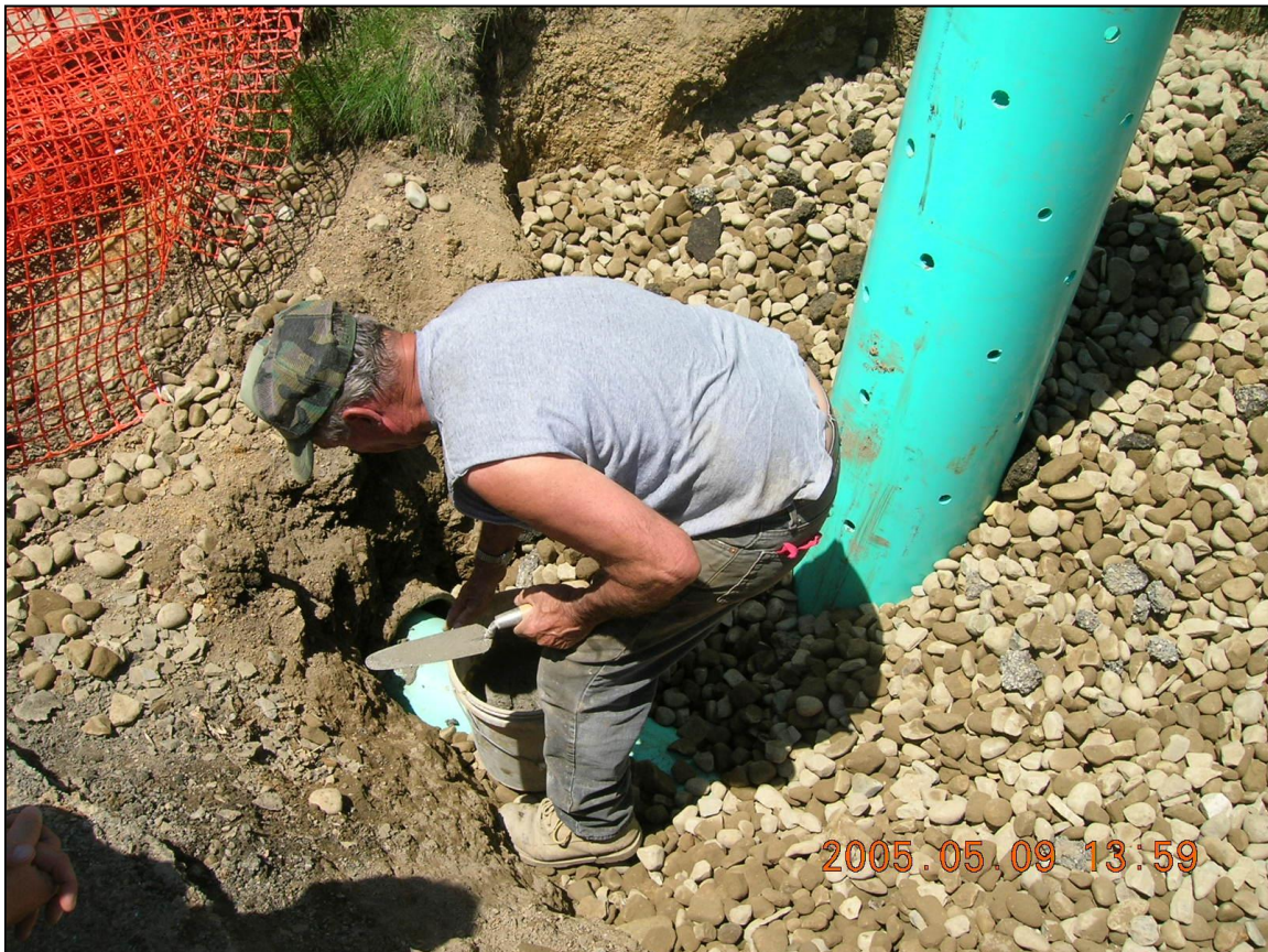
Figure 8. Local resident and subcontractor Dave Menke assists in the installation of the Early Warning System at the “blowout”. (05/09/05)
