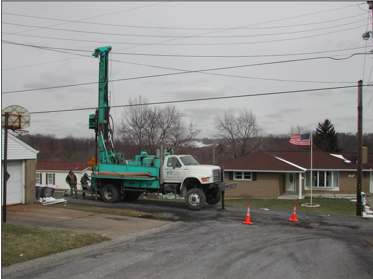
Figure 2. Piezometers installed as part of hydrogeologic investigation. (03/10/05-photo by Rich Beam, BAMR)
