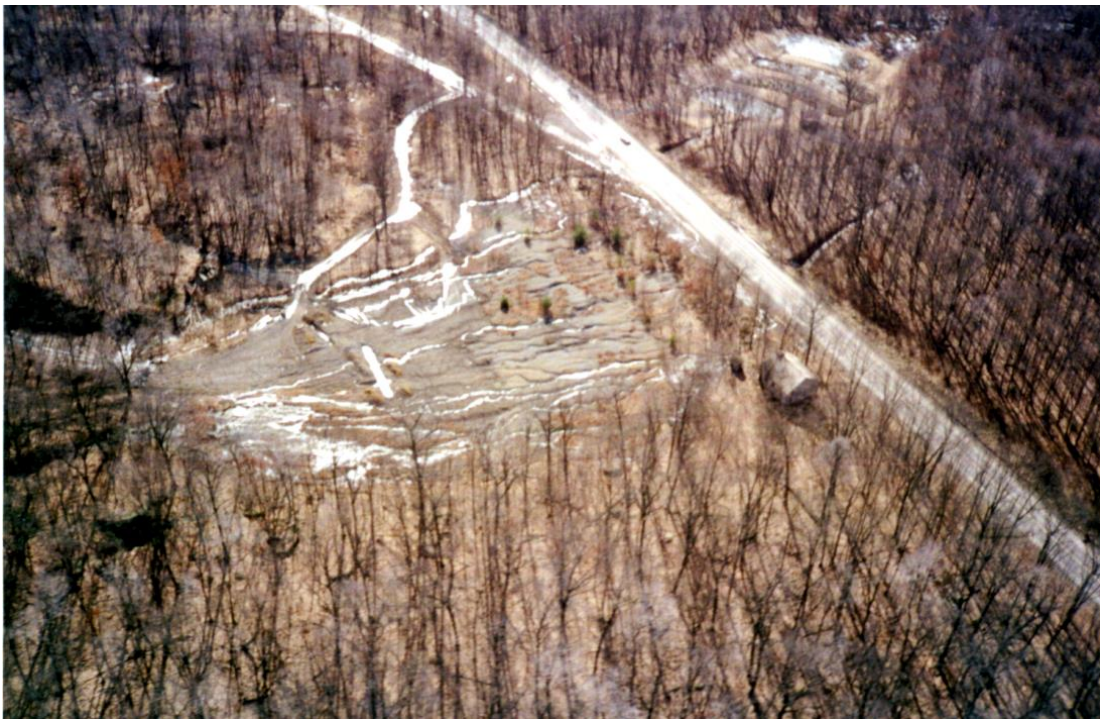
Figure 1. Aerial view (winter 1992); “lower wetland system” (upper right corner); drift entries (center left); area for passive treatment system installation and revegetation (center). (photo by PADEP, Knox District Mining Office)
