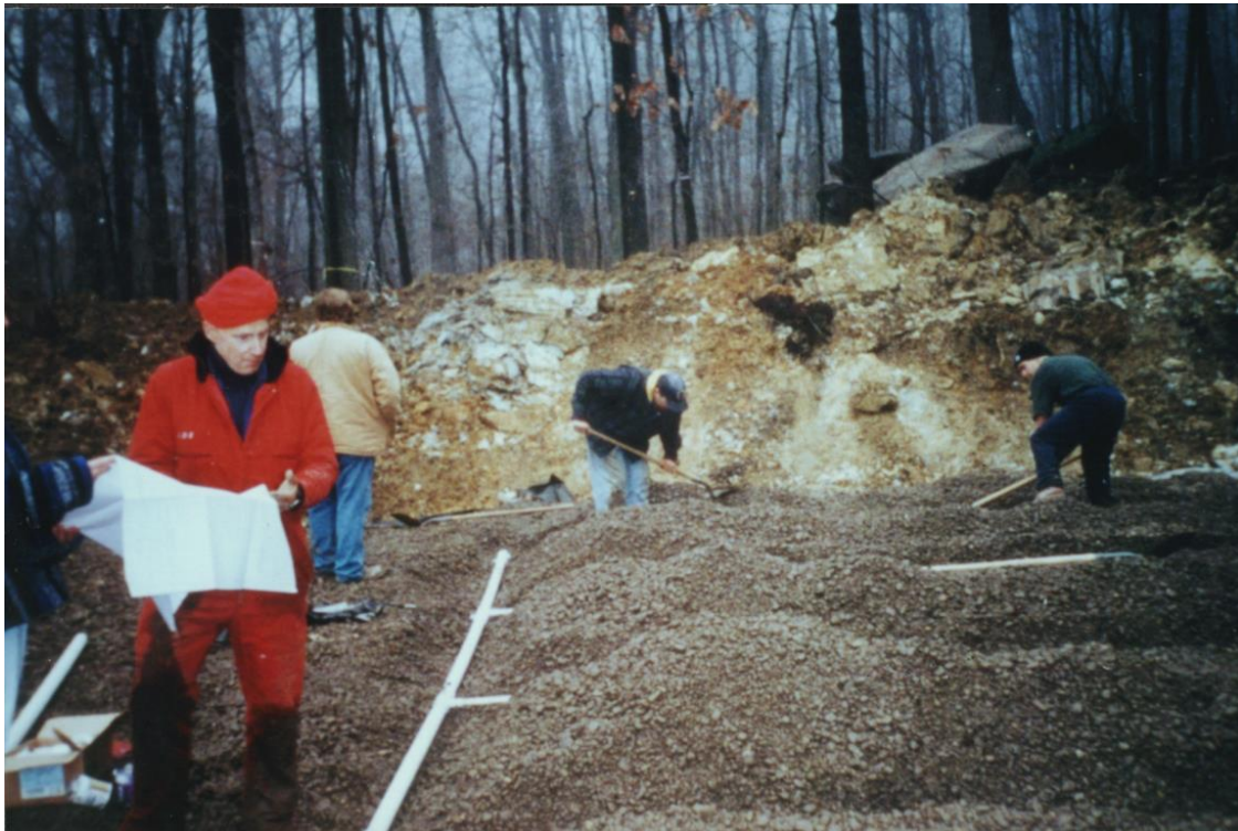
Figure 2. Grove City College and Slippery Rock University students assisting Charles D. Cooper, PE, PLS (CDS Assoc., Inc.) with the installation of the VFP underdrain (1997).
