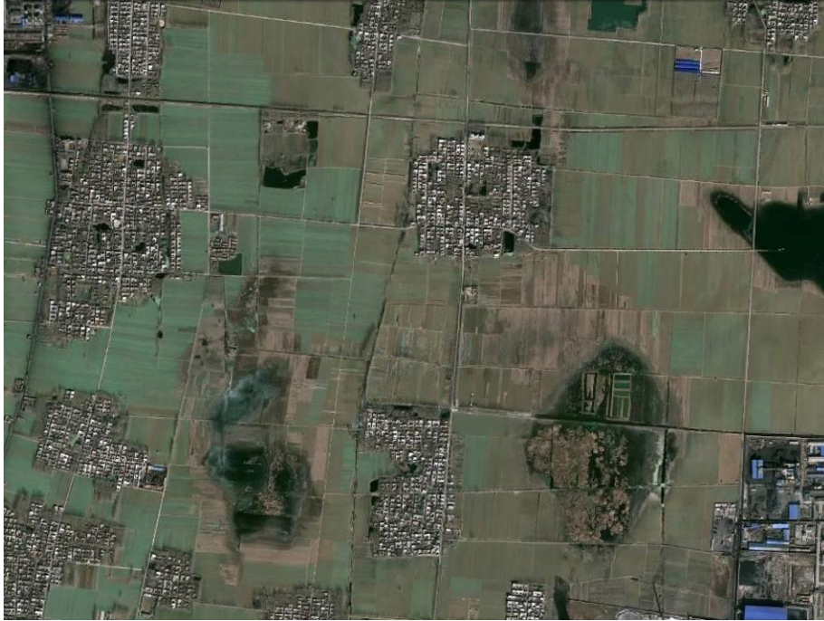
Figure 6. Image from Google Earth showing subsidence impacts near Jining, China.
