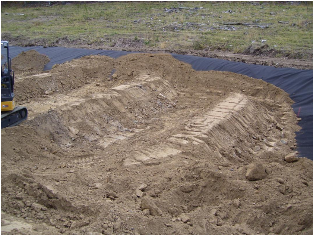
Figure 8. APC earthwork and construction activity.
