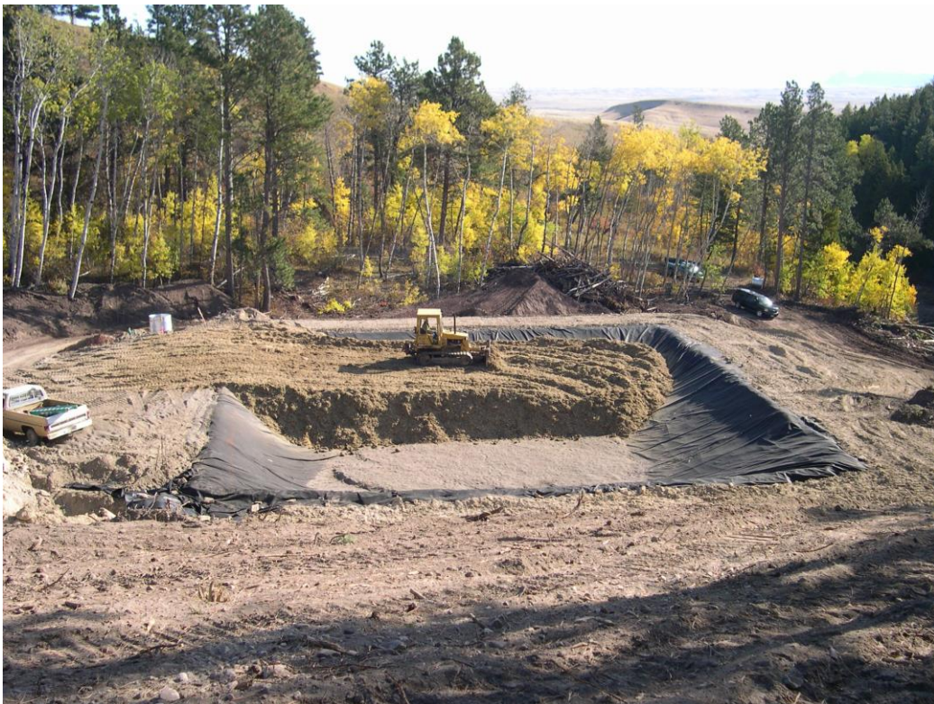
Figure 6. Construction of demonstration-scale BCR; placement of mixed substrate.
