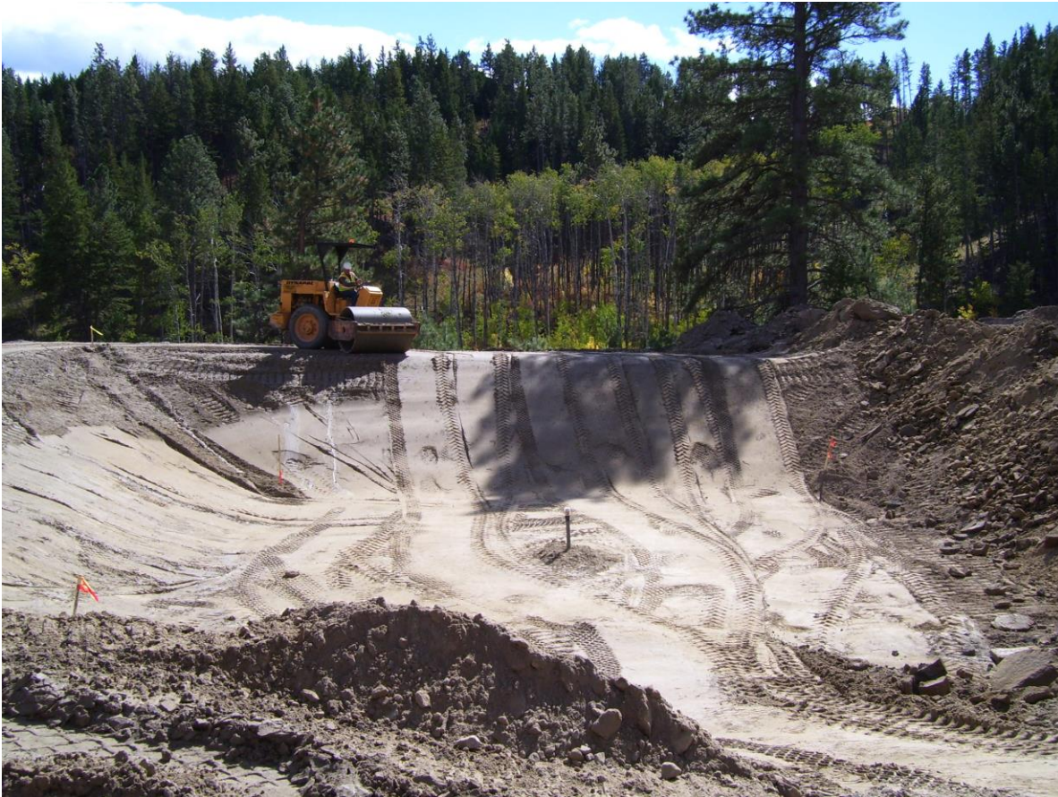
Figure 4. Foundation and compacted fill construction for BCR cell.
