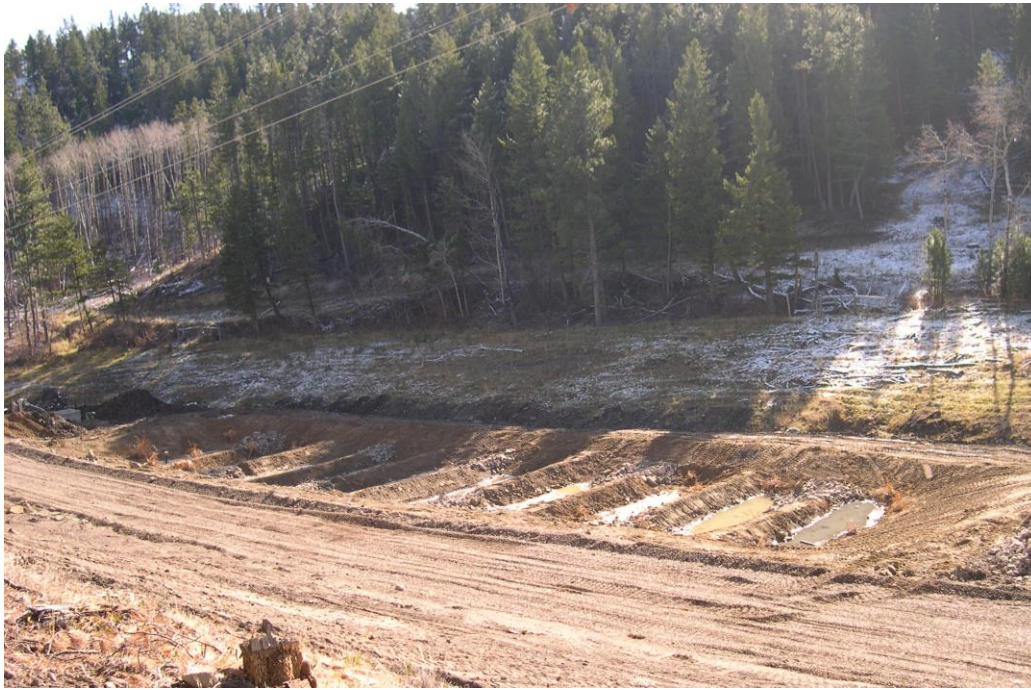
Figure 9. Completed APC, with berms, spillways, and vegetation.
