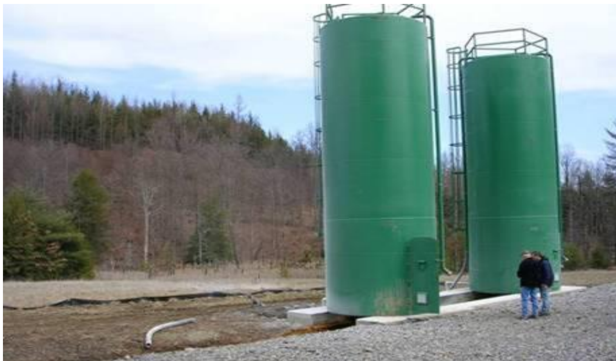
Fig. 20. Lime silos for a tipping bucket lime doser treating another mine discharge in the Porcupine Hollow Tributary of Dents Run.
