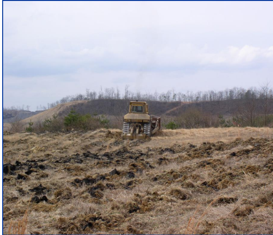
Figure 2. Reclaimed pasture was ripped to alleviate compaction in preparation for tree planting in Knott Co. KY.
