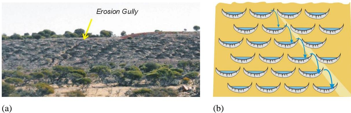
Figure 5. (a) Photograph showing a moonscaped surface on the side of waste rock stockpile with evidence of gully erosion and (b) schematic of the failure mode for most moonscaped surfaces.
