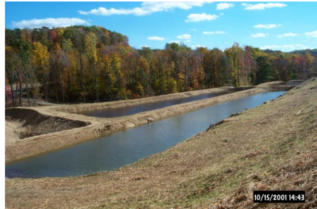
Figure 4: View of flush pond and Vertical Flow Ponds looking south.
