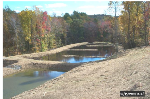
Figure 5: Vertical Flow Pond effluent entering unplanted wetland area to the south. Effluent of wetland enters Laurel Run.
