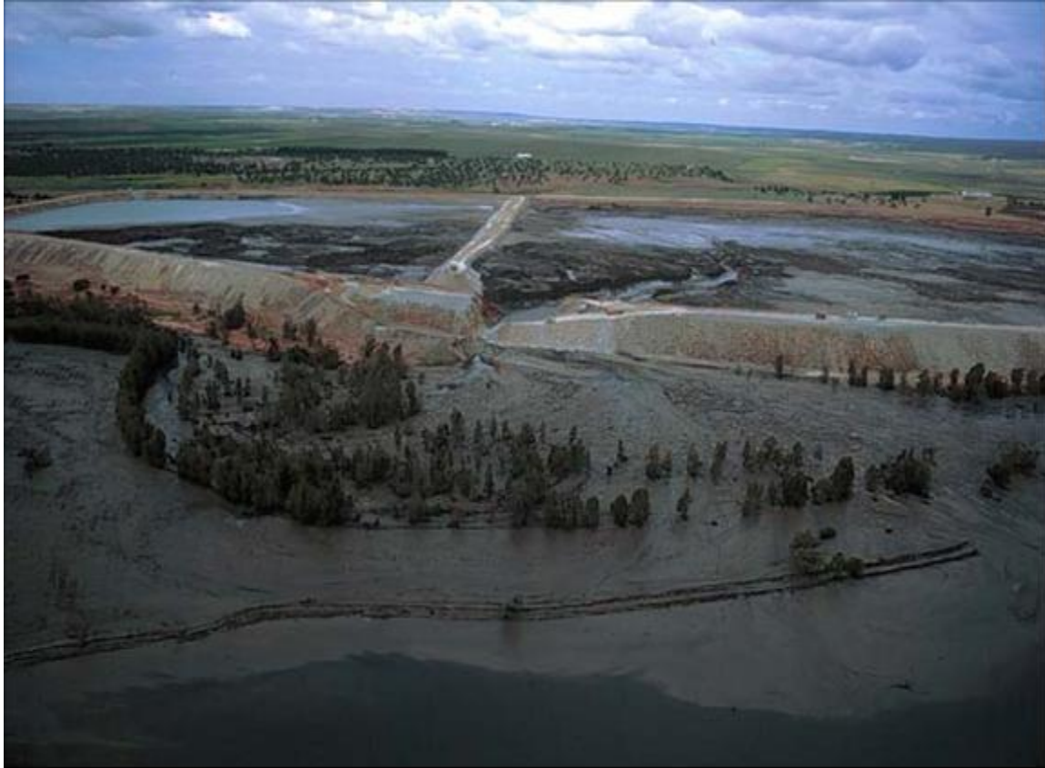
Figure 1. Aznalcóllar tailings dam failure (Photo: Junta de Andalucía)
