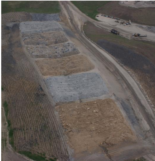
Figure 2. Aerial view of the 2005 loose-dumped plots at the Bent Mountain surface mine in Pike County, Kentucky. The size of each plot is approximately 0.4-hectare.
