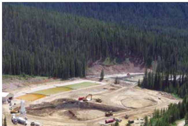
Picture 5. Sediment detention pond.
