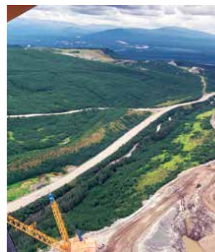
Figure 5. Buttresses were constructed at the base of the slope across the main haul road to support the reclaimed hillside from sliding onto the road and into the creek.
