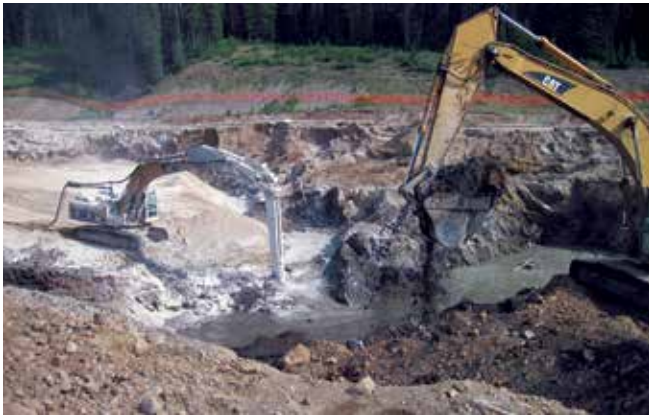
Picture 6. ALLU System placing lime.
