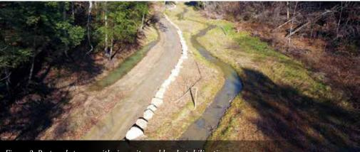
Figure 3. Restored stream with sinuosity and bank stabilization.
