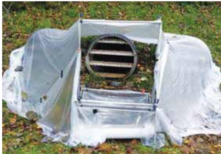
Figure 6. Bat gate attached to culvert with harp trap setup (PHOTO: SANDERS ENVIRONMENTAL).
