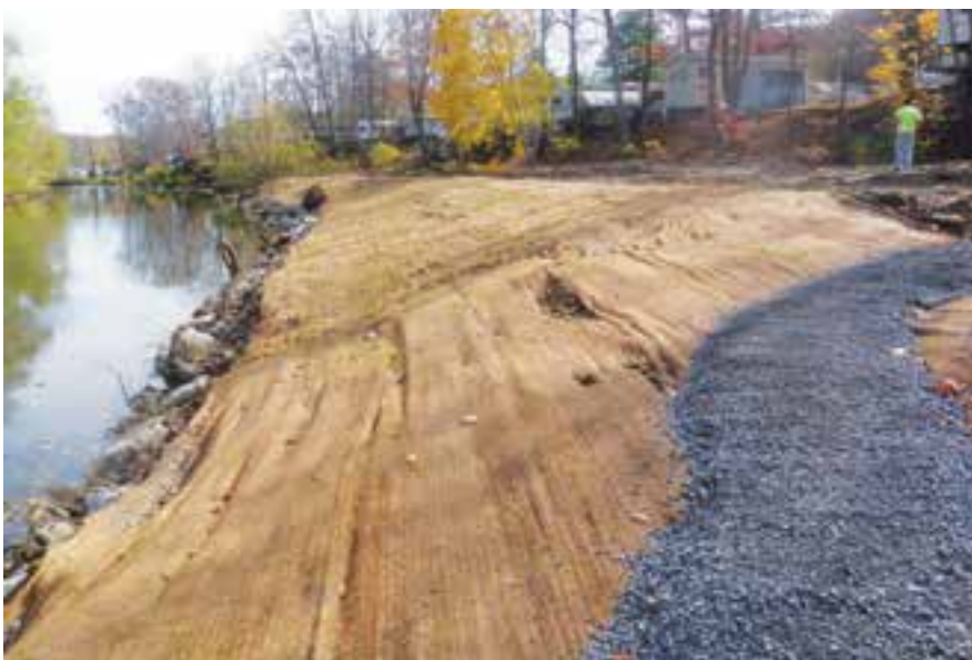
Streambank after construction and prior to tree planting. Grass can be seen emerging through the coconut coir erosion control blanket. One of the four access paths is visible in the foreground.
