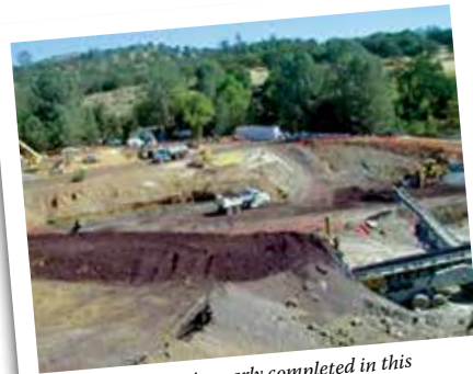
FIGURE 9. The pit is nearly completed in this picture. The oxide tailings (red/purple material in foreground) are being treated and added via the conveyor to the right.
