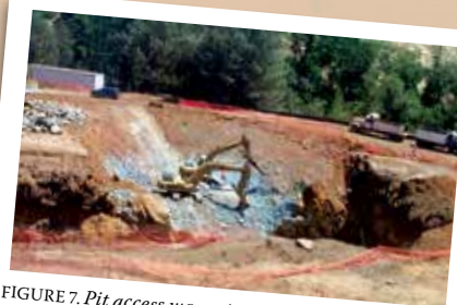
FIGURE 7. Pit access was gained through a ramp constructed on the mine foot wall. After access, a base of crushed limestone rock was added to allow equipment to begin layering incoming treated mine waste.
