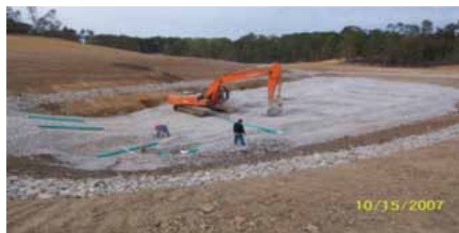
Figure 3. Construction of the Tab-Simco bioreactor cell: limestone-bedded underdrain.
