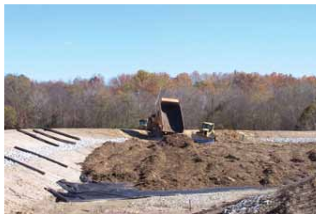
Figure 4. Construction of the Tab-Simco Bioreactor Cell: placement of the compost layer.
