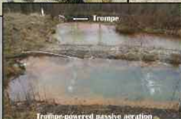
Trompe-powered passive aeration
