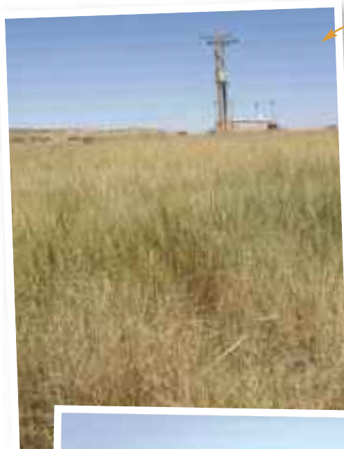
View of header house at Satellite 3-1, Willow Creek ISR U mine site, with typical prairie grass in foreground.
