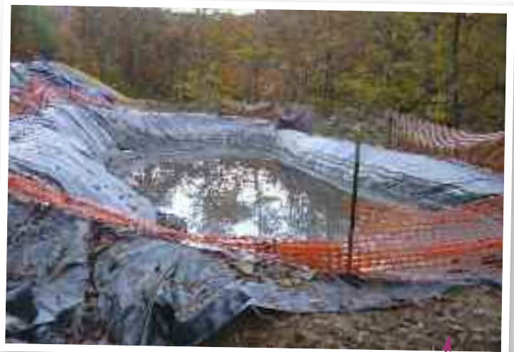
Figure 10. A holding pond lined with a plastic material to store drill cuttings and water at a Marcellus well site.
