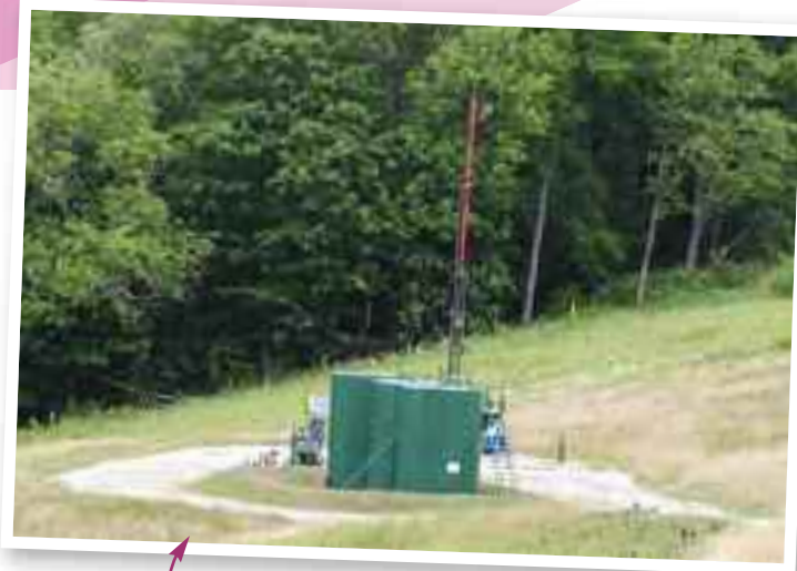
Figure 7. Reclaimed Marcellus Shale drill site showing access road, well head and condensate tank.
