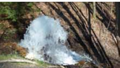
Figure 7. Shawmut portal discharge May 2011.
