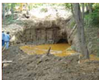
Figure 6. Portal Excavation on September 15, 2009.
