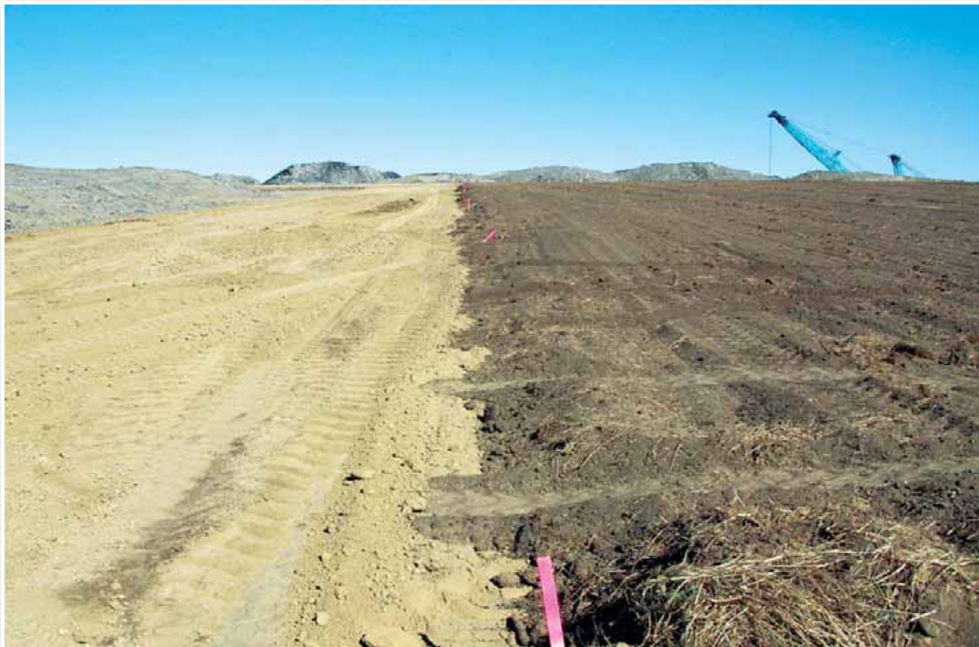
Figure 1. Topsoil is replaced at the BNI Mine near Center, ND. Topsoil salvage and replacement on the land surface provides for agriculture post-mining land uses.
