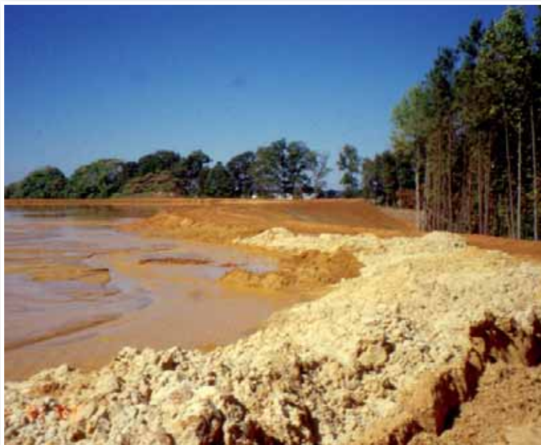
Figure 3. Dewatering tailings and slimes at Old Hickory Project. The light colored dike material in the foreground is topsoil that is forming a section of the enclosing dike wall. Once the surface of this pit has dewatered sufficiently, it will be limed, fertilized, and deep ripped to prepare it for revegetation. Significant swell in the slimes often results in a final elevation above the pre-mined lands, which complicated topsoil return during the early years of mining. Later mining operations have kept topsoil berms isolated away from enclosing mine pit dikes.
